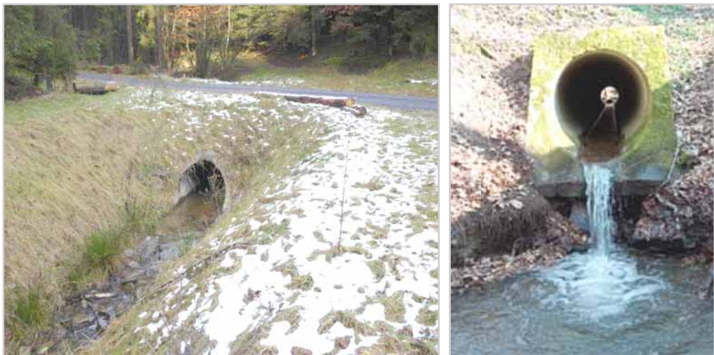
Fig. 4.4-13: The culvert on the left under the stream crossing has sufficient depth of cover and stream bed substrate; the culvert on the right is an impassable barrier for aquatic fauna (photos: Peter; Thomas)
